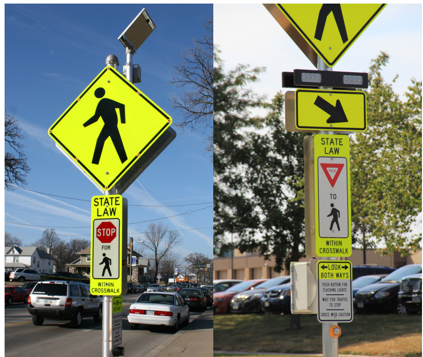
LEDs around crossing sign border (left) and RRFB under sign (right)
