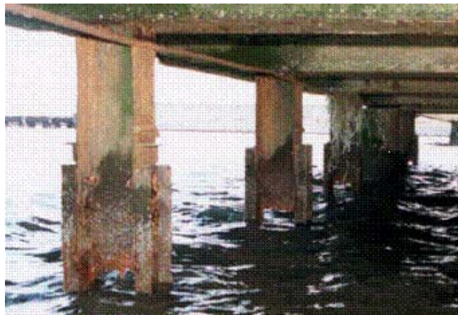
Figure 1.8. Corroded steel piles with loss of section in a marine environment (Juran and Komornik 2006)
