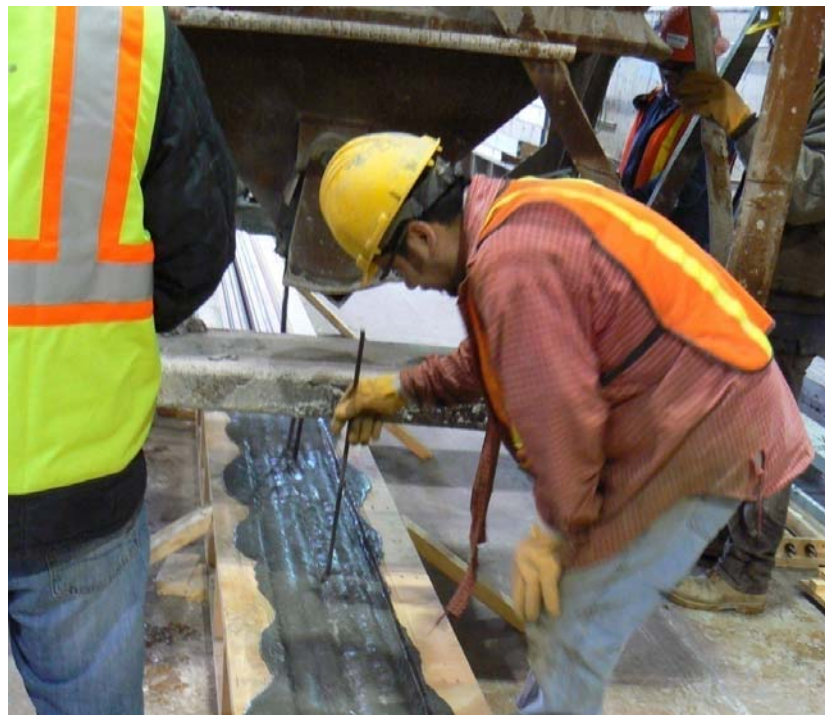
Figure 4.24. “Rodding” through the web of UHPC to eliminate formation of possible air pockets
