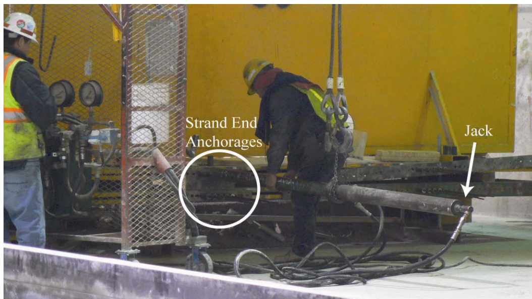
Figure 4.12. Stressing of prestressing strands for UHPC pile P1
