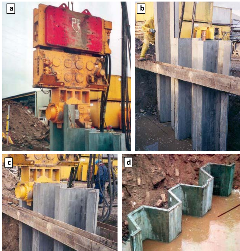
Figure 2.44. Views of a) to c) the driving process for SCFRC sheet piles and d) the completed view (Walraven 2007, Walraven and Schumacher 2005)
