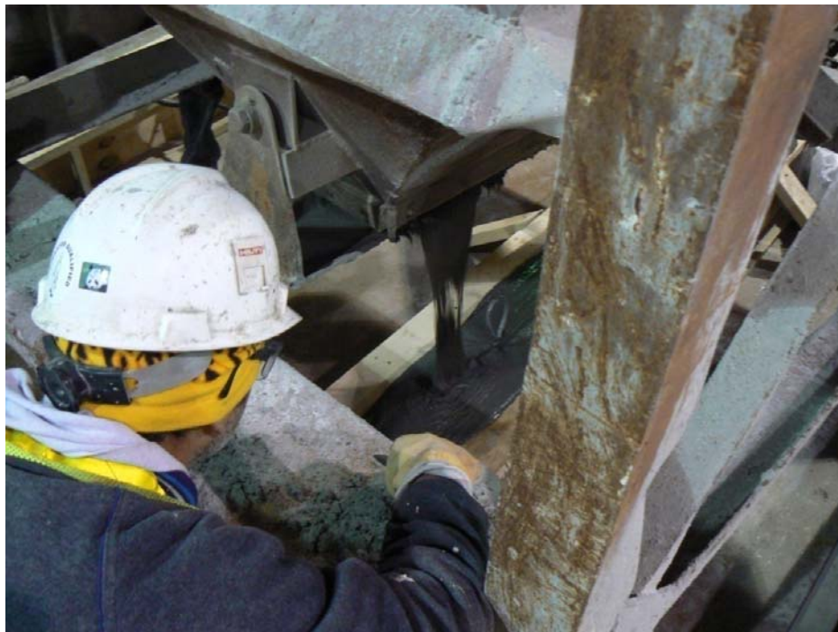
Figure 4.18. Beginning of first pour of UHPC units
